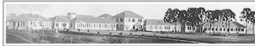
Detalhe 1 Pavilhão Principal Hospital
